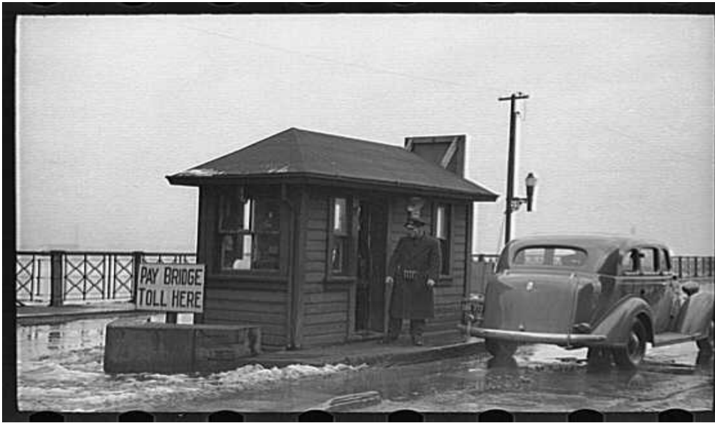
Figure 1 Toll Bridge across Mississippi River at St. Louis
